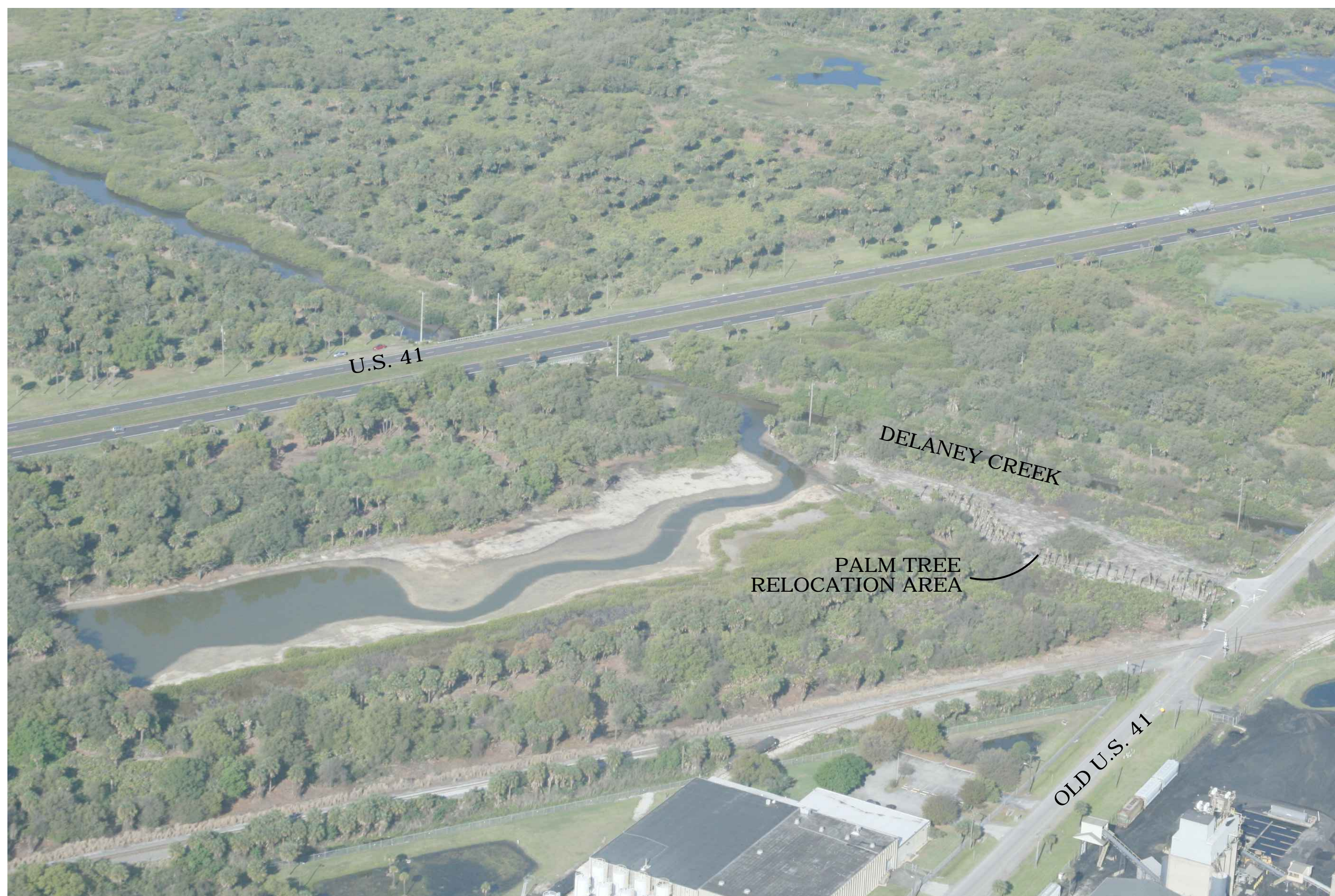
BORROW PIT RESTORATION SITE (03-15-2014)
