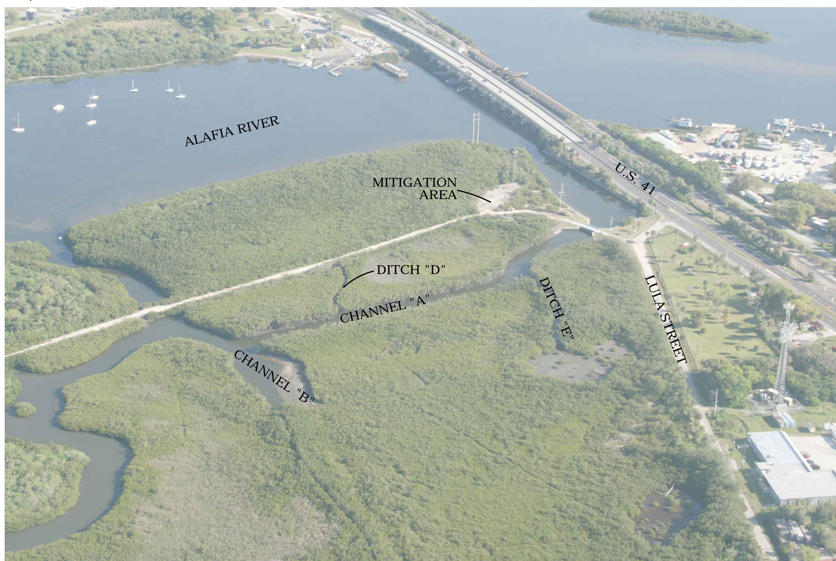
GIANT'S CAMP OVERALL RESTORATION (03-15-2014)
